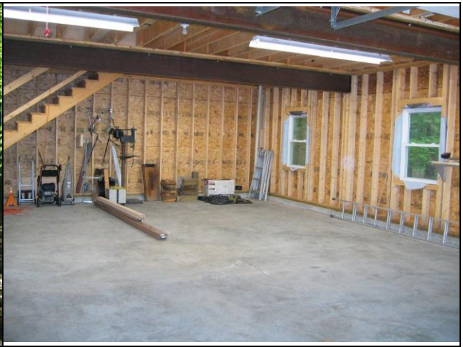
Four Car Garage: 200 Amp service, Trussed Roof, High intensity lights – 2 zones, Open 2 nd floor, 2 X 6 inch walls, Steel beams – no central columns, ~ 1800 sq. feet (2 floors)
